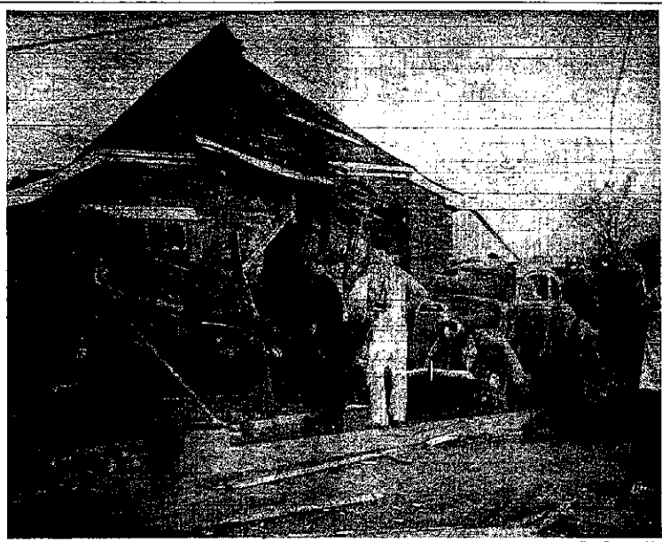
Wreckage of the Western Illinois Oil Company's filling station, 2709 West Main Street, following yesterday's tornado. The car setting upright in front of the door is the one in which Joseph Roesch, former president of the Roesch Enamel Range Company, was riding when the twister struck the machine and hurled it against the station. Roesch was crushed to death. The picture was taken a moment after Roesch's body had been removed and less than 30 minutes after the tornado had struck.
